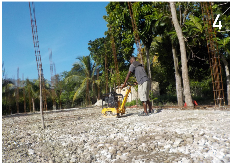
In late August, the final load of small stone is added and compacted in preparation for the pouring of the cement floor.
