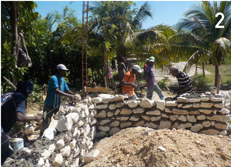
Stone foundation of first wing is completed by hand in early August, employing over 40 Haitian craftsmen.
