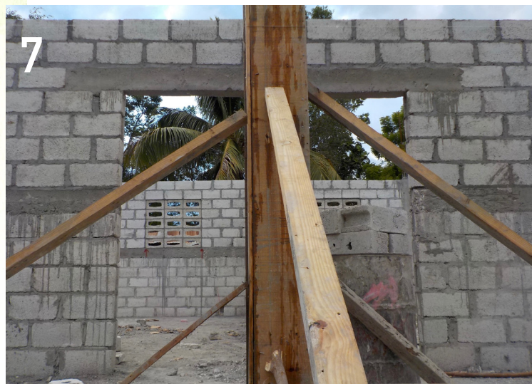
Walls are completed in early November and portico beams are framed and ready for pouring.
