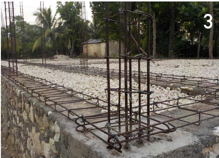
Rebar and gravel prepare the foundation for pouring of the cement floor.
