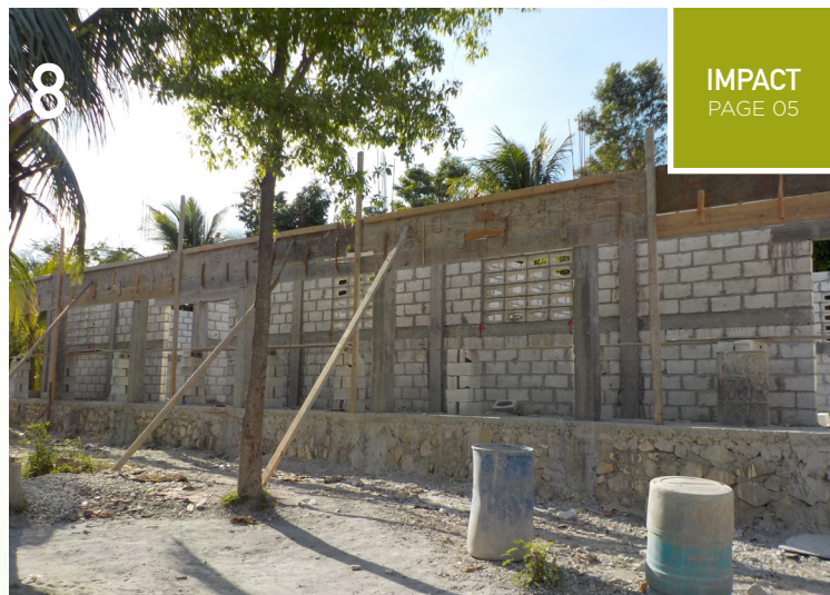
By mid-November, the header between the portico beams is framed. Once poured with concrete, this will help support the roof.
