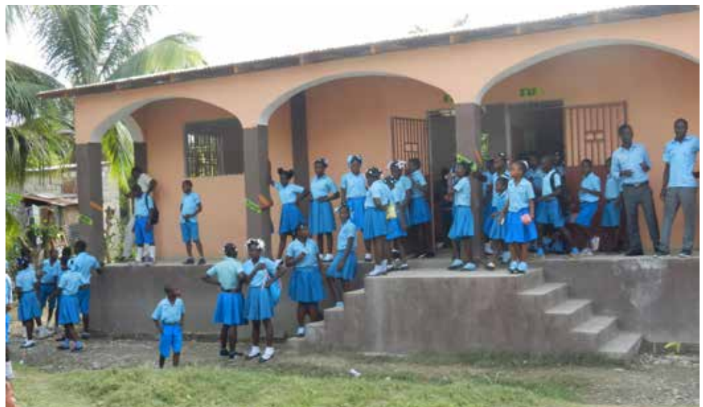
Students exiting 2 of the 8 classrooms at the newly constructed school in Desarmes, Haiti
