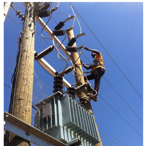
New transformer being installed
