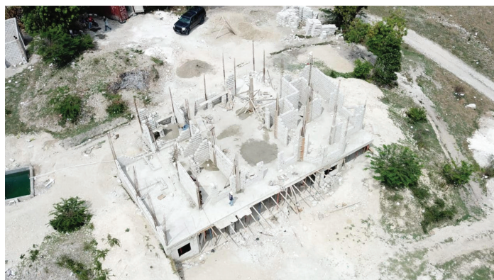
April 2021-Second floor walls are underway. Large cistern is installed.
